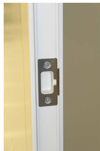
Rounded part of the lock is easier to clean
